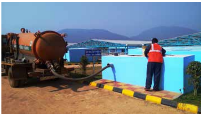
Figure 17: Operation of FSTP Dhenkanal
